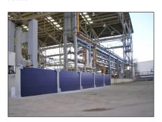
Multi-span 900mm high removable containment barrier.
