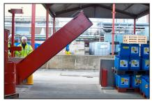
Gas-lift pivot barrier for vehicle access.
